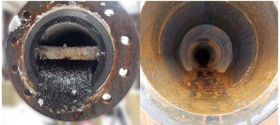
With the client's facility having been decommissioned for more than a year, residual emulsion on internals made for a very sticky situation that traditionally requires mechanical removal. The combination of piping and equipment necessitates methods such as hydromilling, vessel entry and steaming that would prove to be too costly and excessively time consuming.
